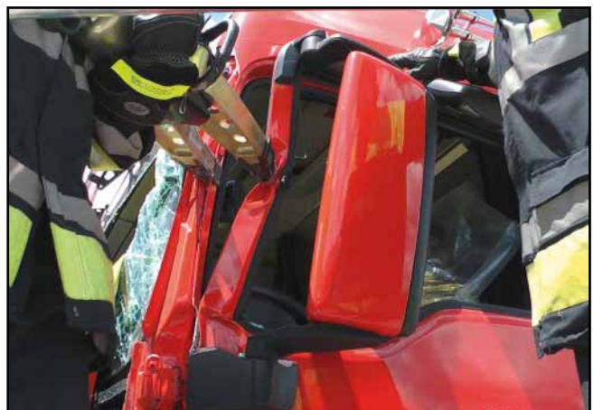
Spreading apart the top of the door
