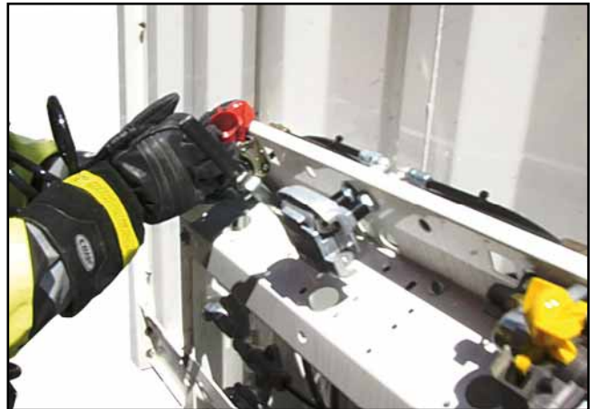
Disconnecting supply lines
