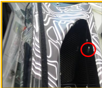
Exterior door release ( WEAR INSULATING GLOVES )
